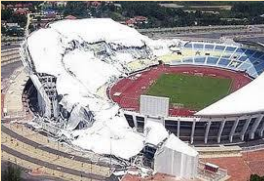
Collapse of Stadium Sultan Mizan, Terengganu in 2008
