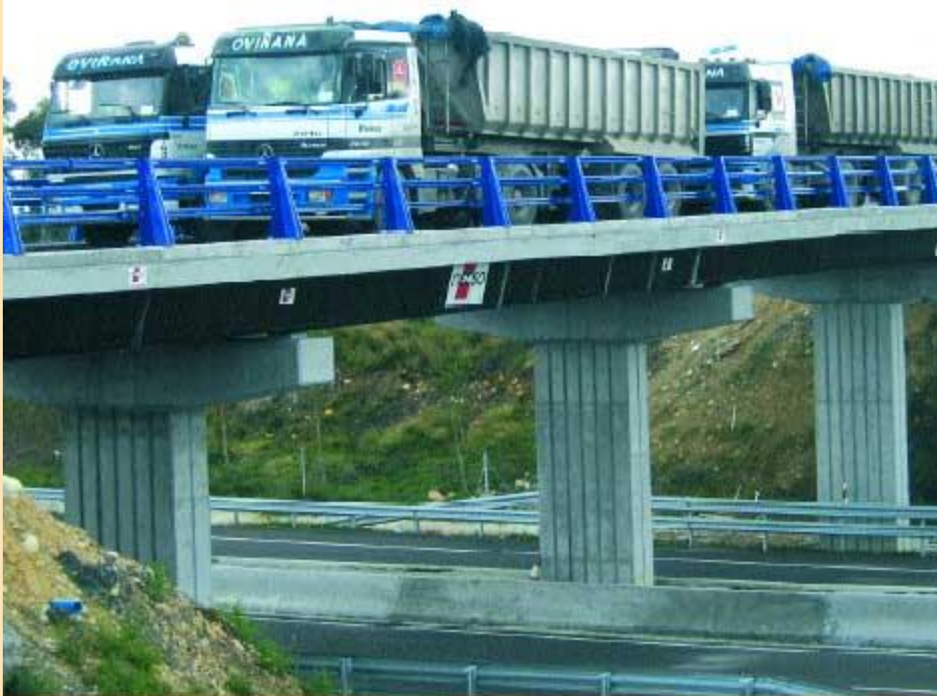
Bridge undergoing load testing.
