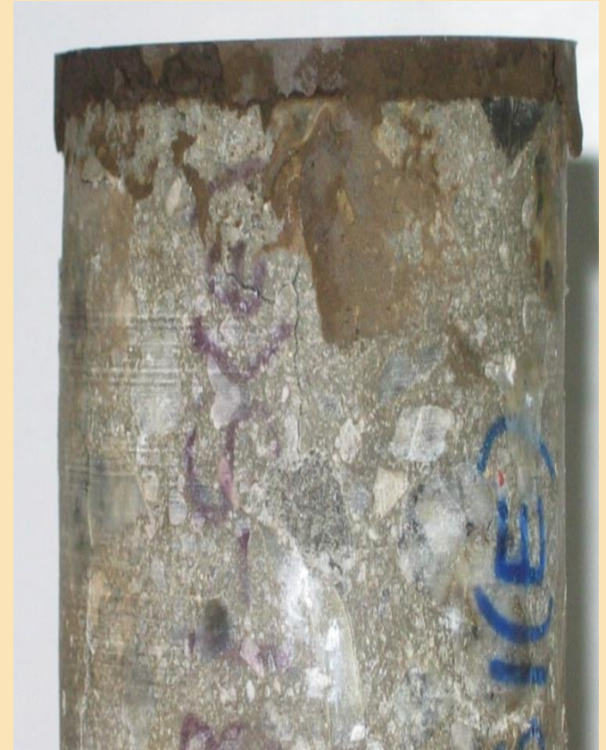
Failure mode of core observed after test
